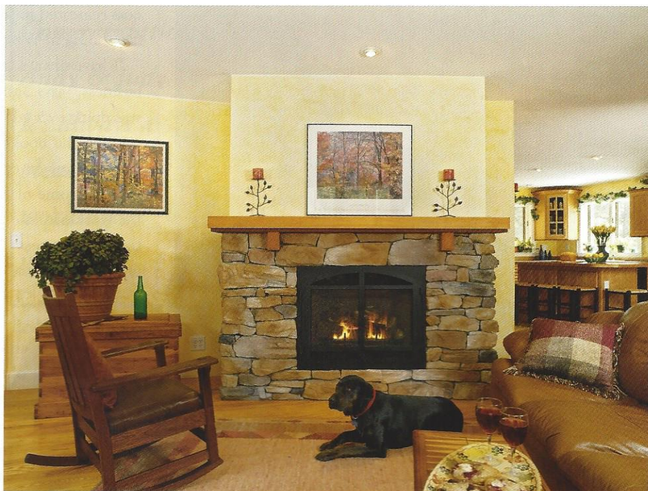
Stepping into the living room, a Mendota gas-fired unit is surrounded by a cultured stone fireplace built by Andy Leach, topped by a mantel he milled from a 100-year-old fir beam salvaged from a previous jobsite. The Eldorado cultured stone was supplied by Cleary Stone Company.
