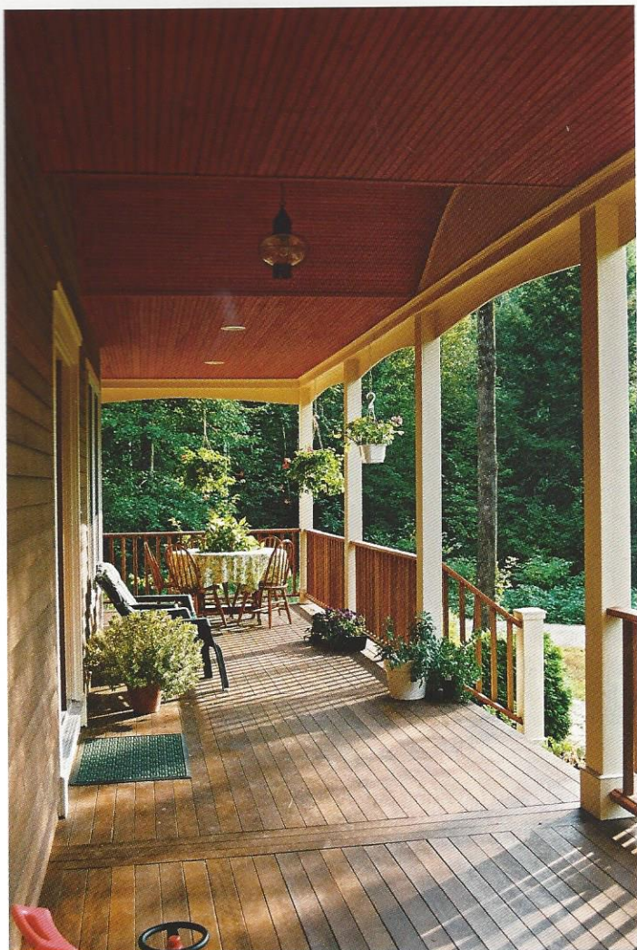
Like a traditional Vermont farmhouse, the Leach home includes an inviting front porch, with built-in barrel vault ceiling, custom trim details and custom-milled fir handrails and posts, all by Leach Construction. The southern yellow pine beaded ceiling and mahogany decking are both from Milton Building Supply.
